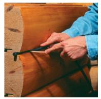
1. Install backer rod into the caulk well of clean, stained logs.
